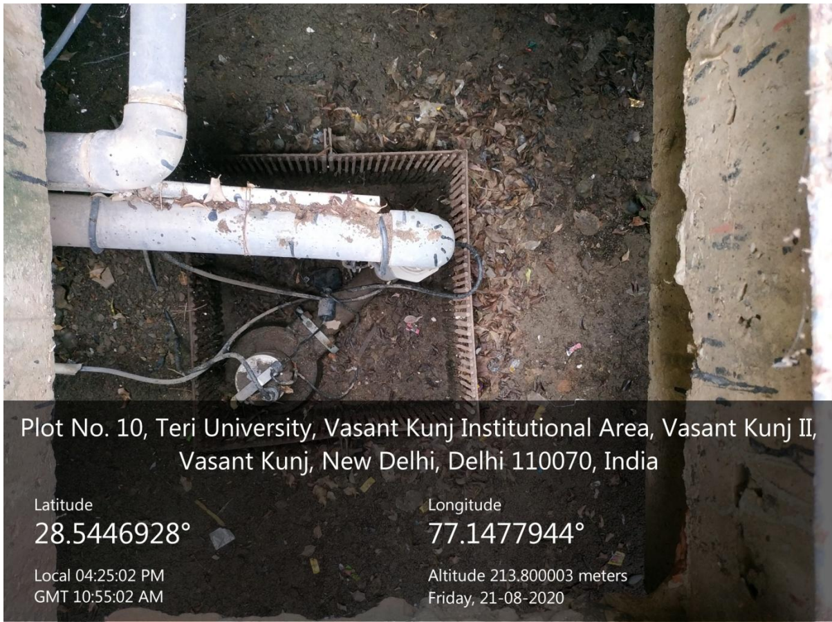
Geotagged photo of Rainwater Harvesting Facility in the TERI SAS campus
