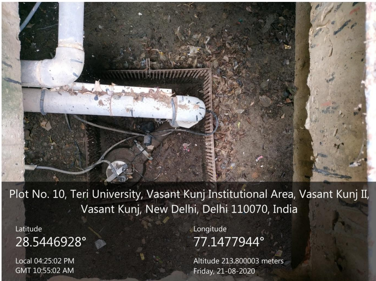
Geotagged photo of rain water harvesting in TERI SAS campus
