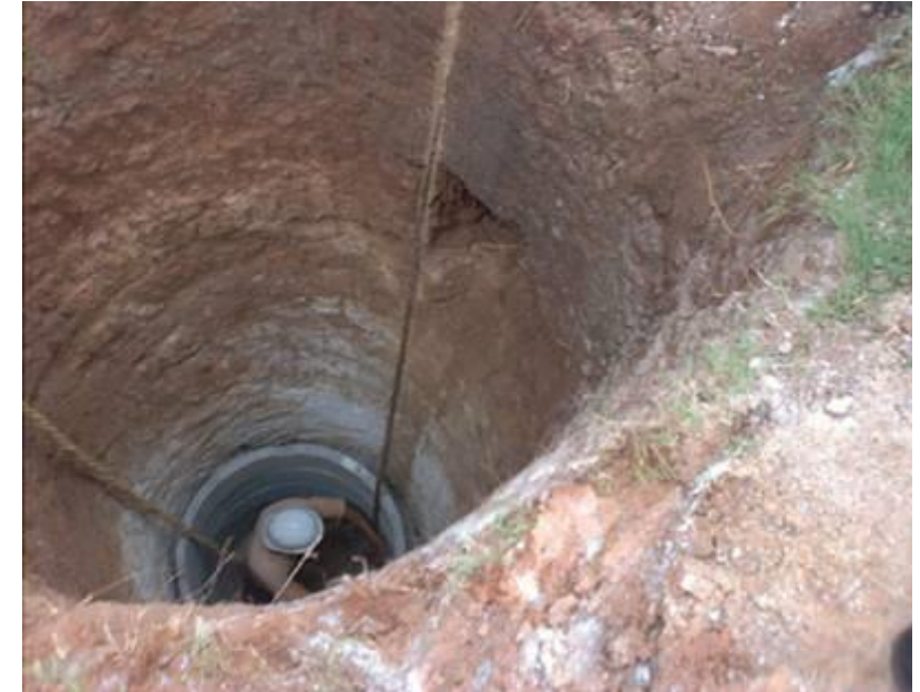
Placing of the rings
