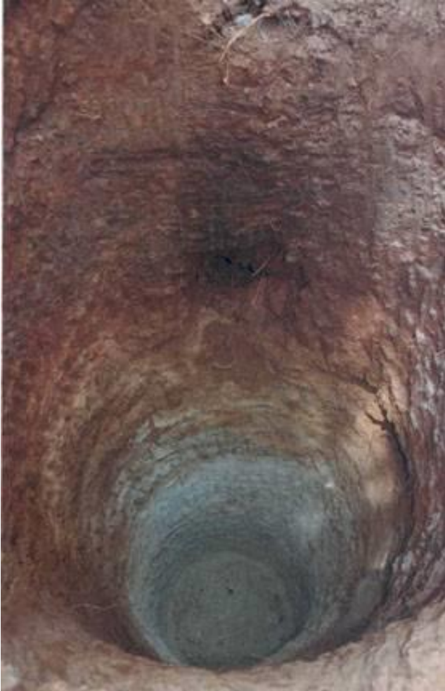
The pit has reach the silt layer
