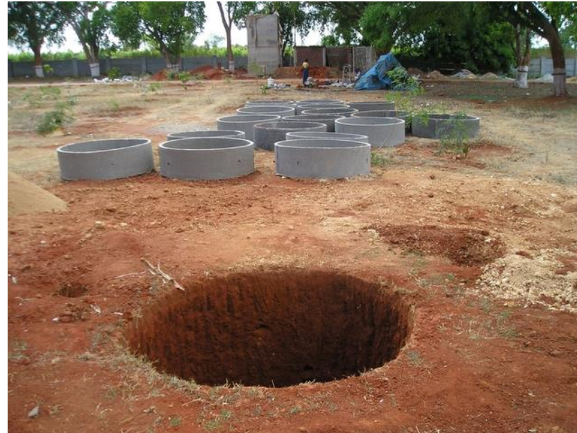
Pit and concrete rings
